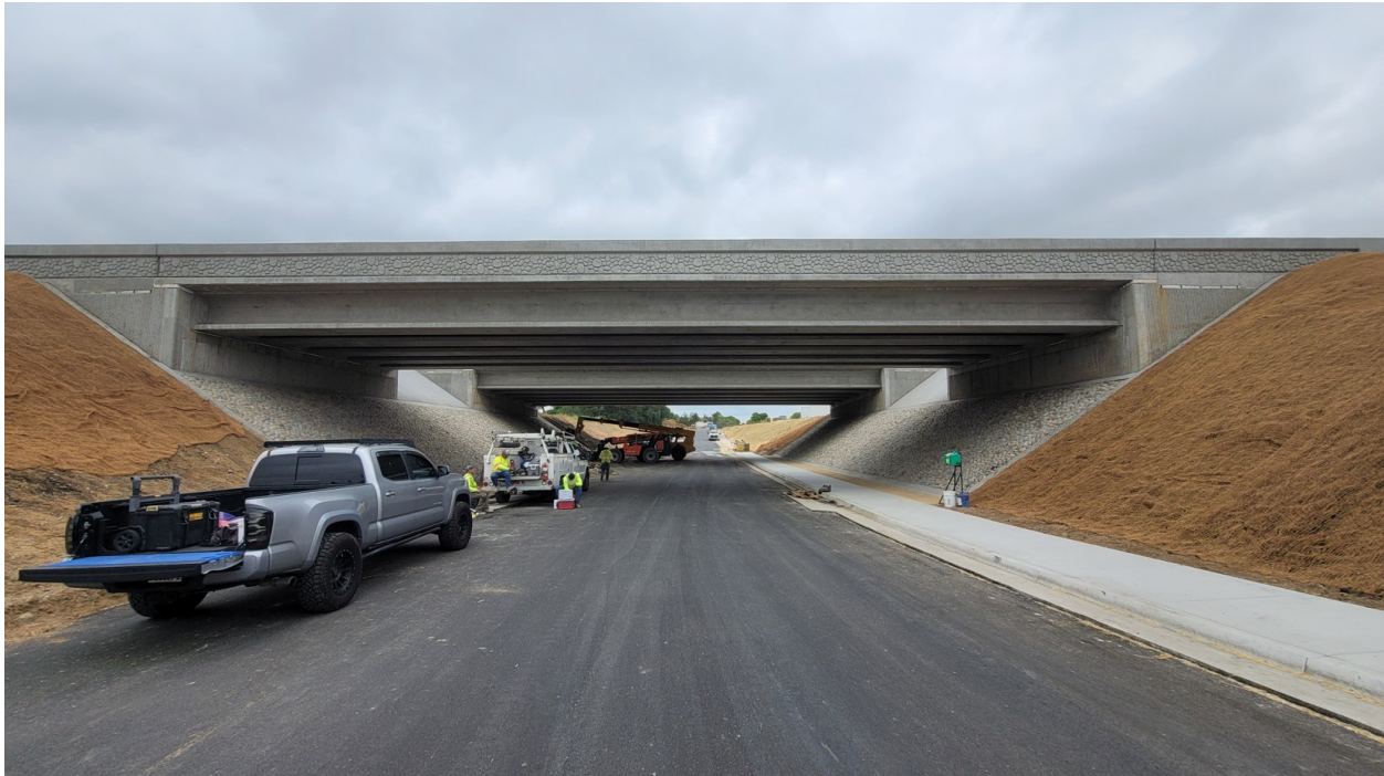
Photo of new undercrossing, under US 101 south of Wellsona Road.
